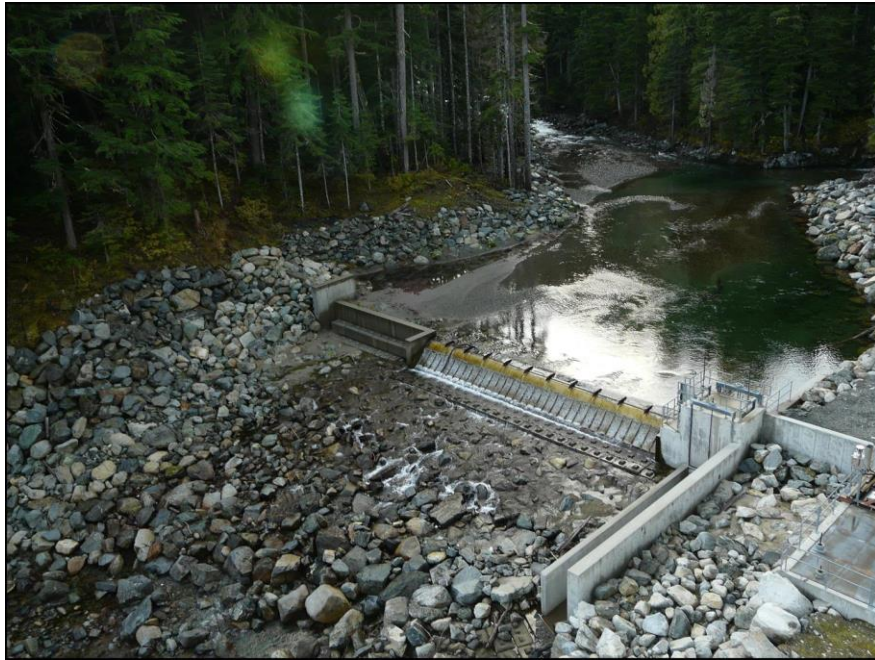
Figure 3-24: Typical Coanda intake
